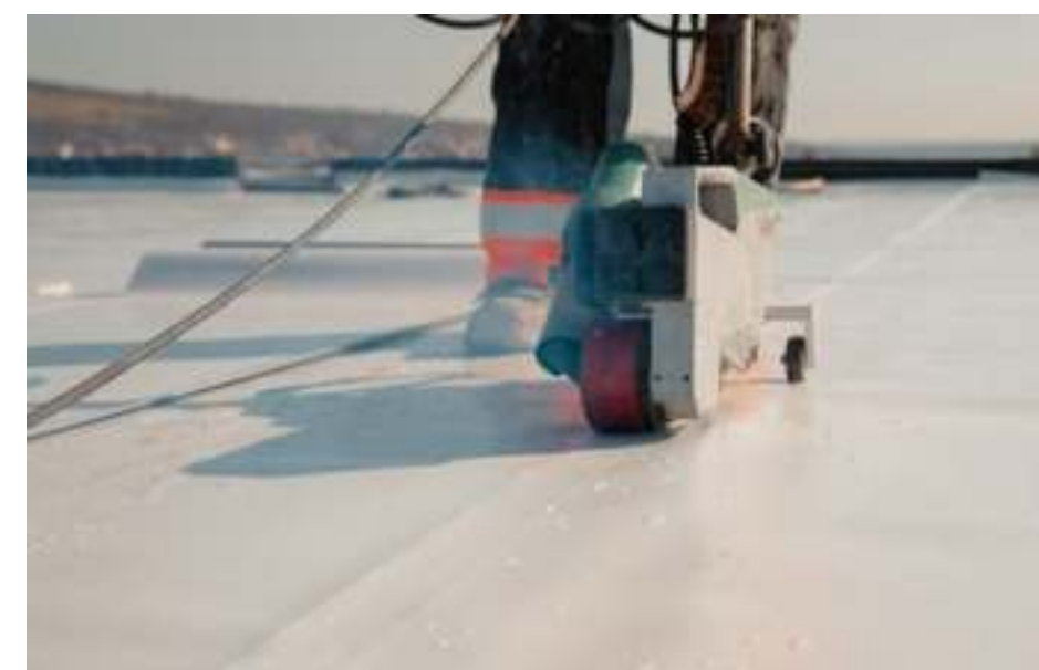
Thermoplastic polyolefin roof
